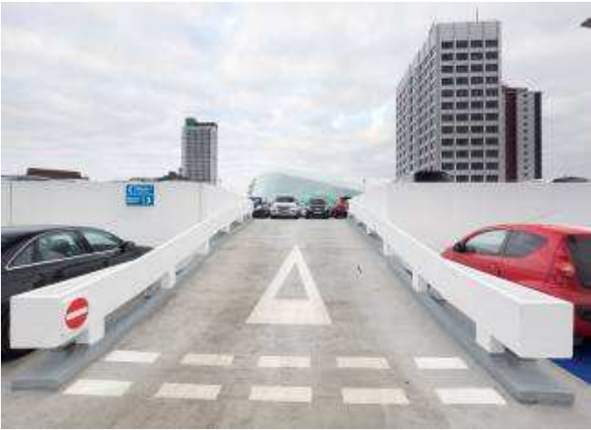
Full top deck coating & parking pads to Gade
